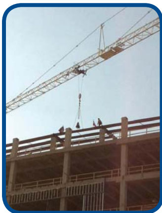
The final "signed" steel beam was put in place on October 27.
