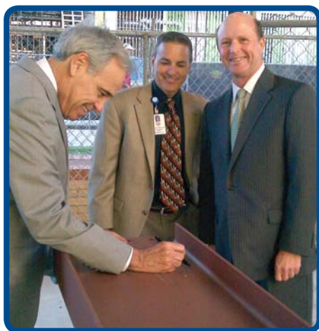
(On left) U.S. Congressman Charles Gonzalez, Dist. 20, signs the final beam, as Sergio Farrell, VP, Ambulatory Services and Mark Webb, VP, Facilities Development & Project Management look on.
